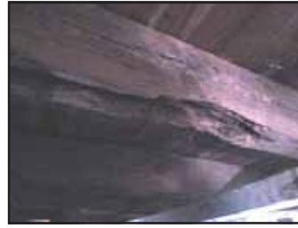
Damage to floor of sunroom
