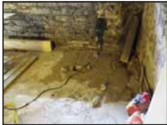
Temporary supports going up in basement
