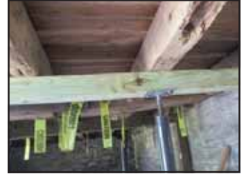
Damage to floor of sunroom
